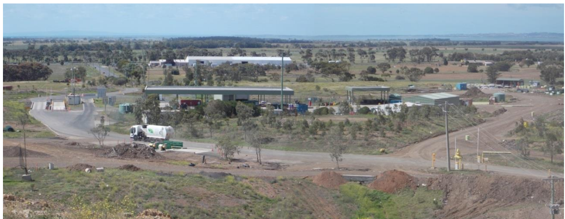
Figure 4 Transfer Station and weighbridge
