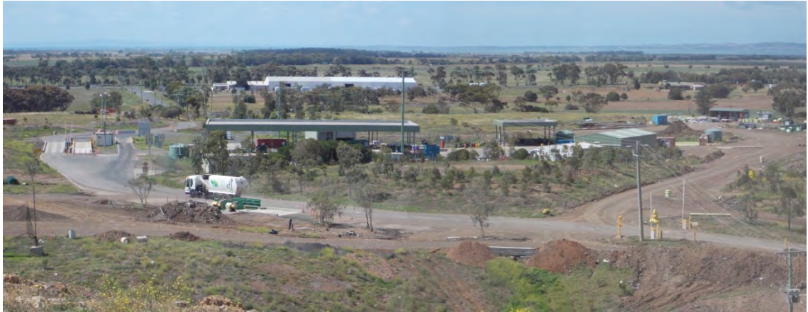
Figure 5 Transfer station and weighbridge
