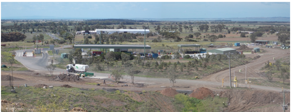
Figure 5 Transfer station and weighbridge
