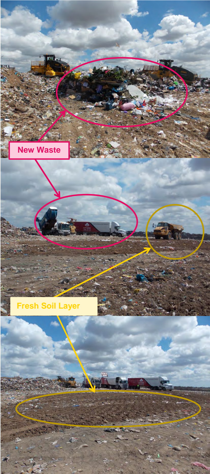
Figure 18 Active landfill tipping face
