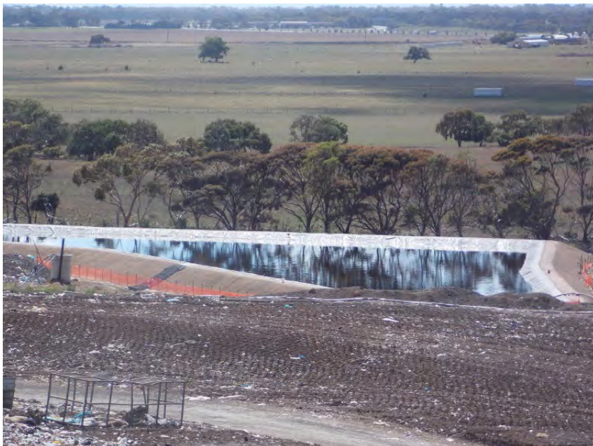
Figure 12 Newly constructed east leachate pond
